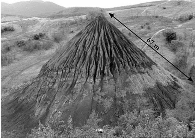
FIG. 3 - The surface of the younger, northeastern cone with a slump zone in the middle. By now this zone has completely shifted to the top in the case of the older cone.
