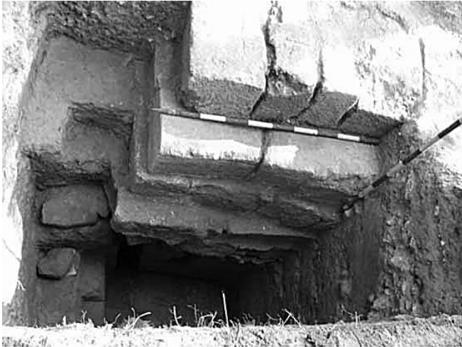
FIG. 6 - Detail of the massive masonry walls, with large hand carved limestone bricks.
