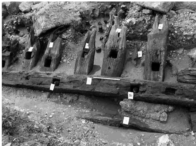
FIG. 5 - A unique well preserved structure of the fortress basement made by intricate oak trunks grid on the Danube muddy riverbed.
